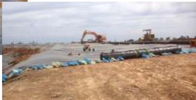
*SITA staff were required to sandbag the edges of the liner during the installation process.*
